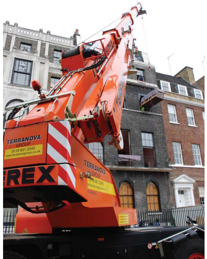
The crane in action
